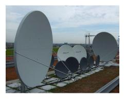
Additional satellite services can be added to an IRS by providing more satellites dishes at the head end and more backbone cabling and equipment to distribute the extra signals.
